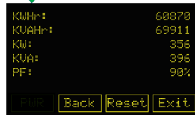
Power Metering Screen
